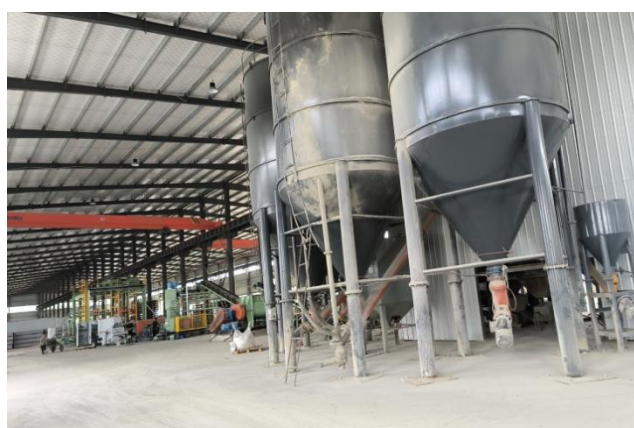
轻质水泥隔音板车间
